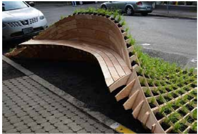
Figure 25 Lattice shell structure
